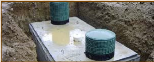
Individual wastewater system septic tank
