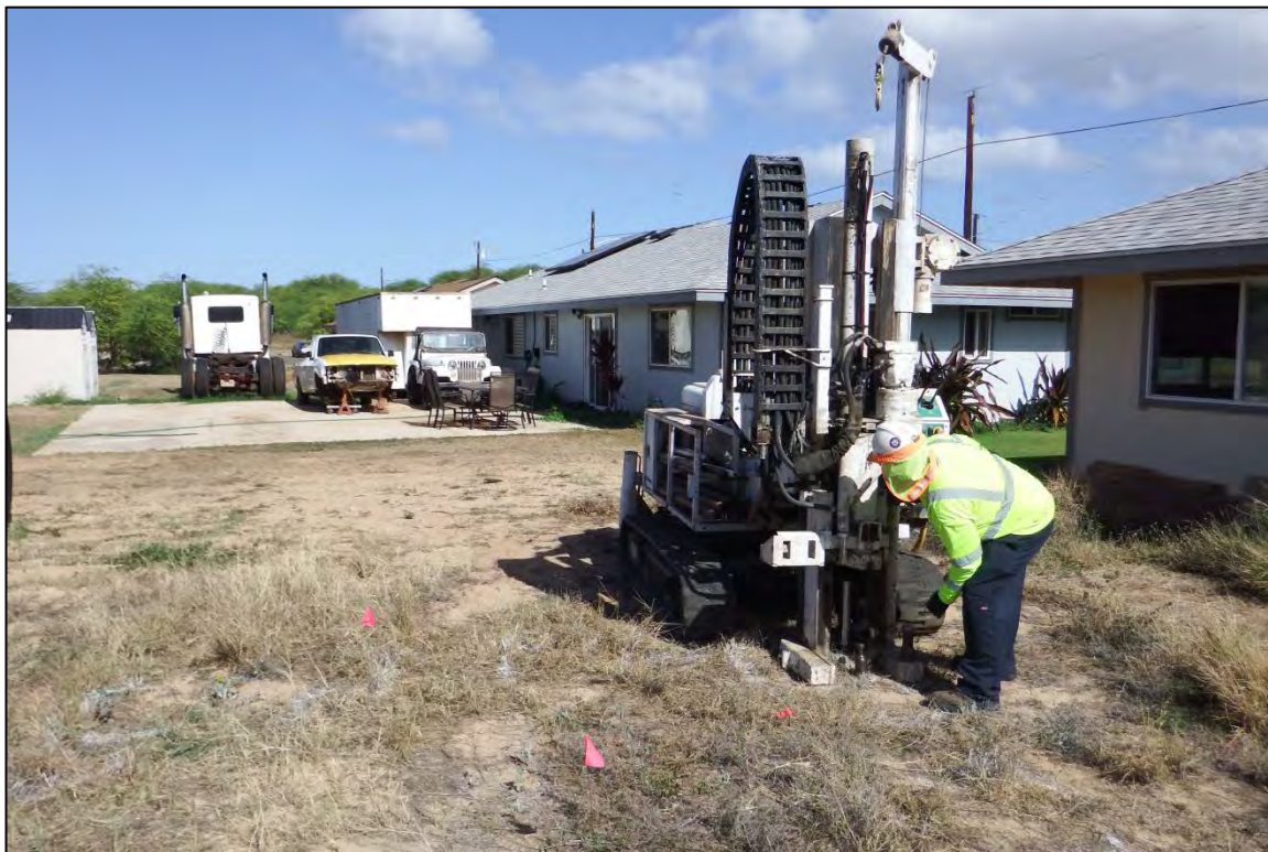
Photograph 31: Typical photograph showing direct push borings in progress.
