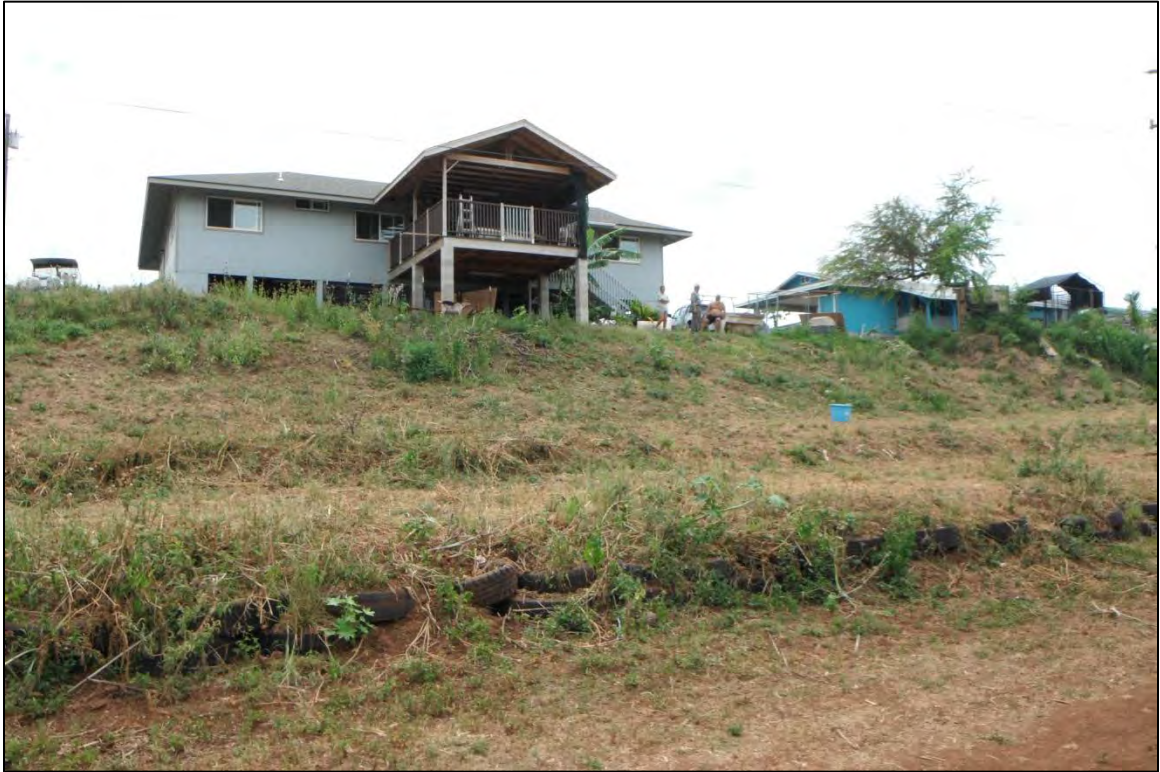
Photograph 20: North slope of Lot 3 in DU1. View from Cane Haul Road.
