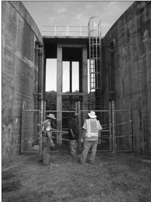
Figure 85. Entryway and ladder separating the two 3.5 MG tanks.
