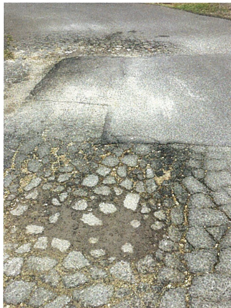
Photo 2.8. Potholes and Cracking on Parking Lot
