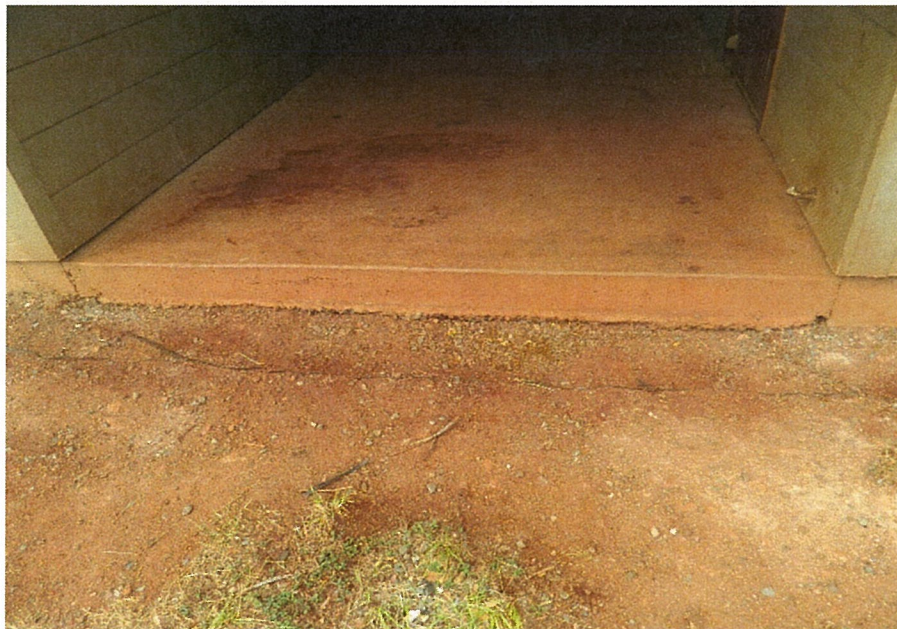
Photo 3.11. Exposed Slab
