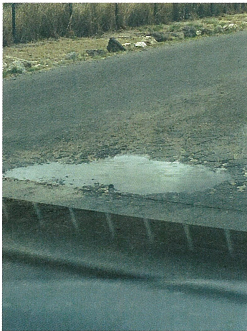
Photo 2.1. Holt Road, Asphalt Concrete Depression
