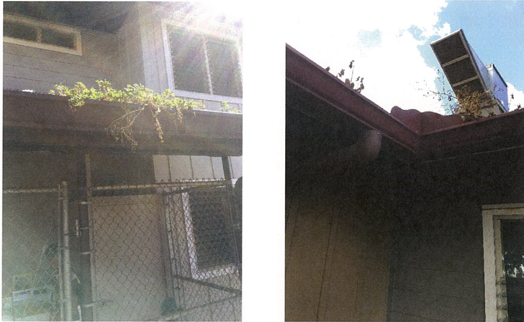
Photo 2.5. Debris in Gutters
