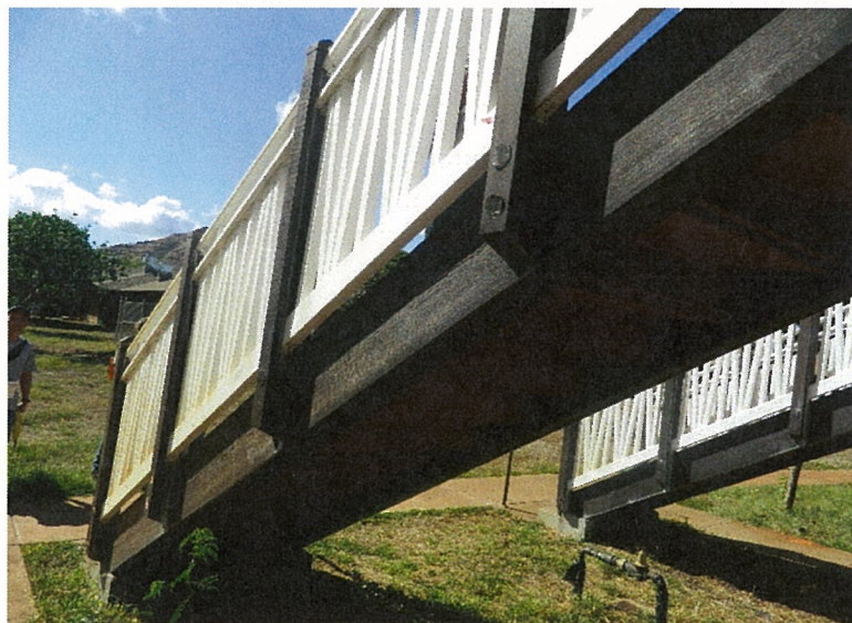
Photo 3.3. Wood Railings Bolted Outside
