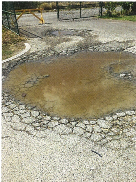
Photo 2.8. Potholes and Cracking on Parking Lot
