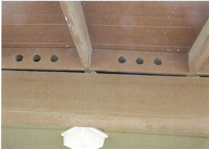
Photo 3.12. Roof Beam Gap
