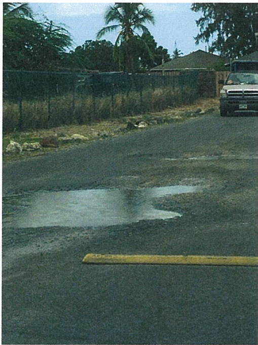
Photo 2.1. Holt Road, Asphalt Concrete Depression
