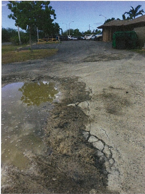
Photo 2.7. Ponding on Driveway
