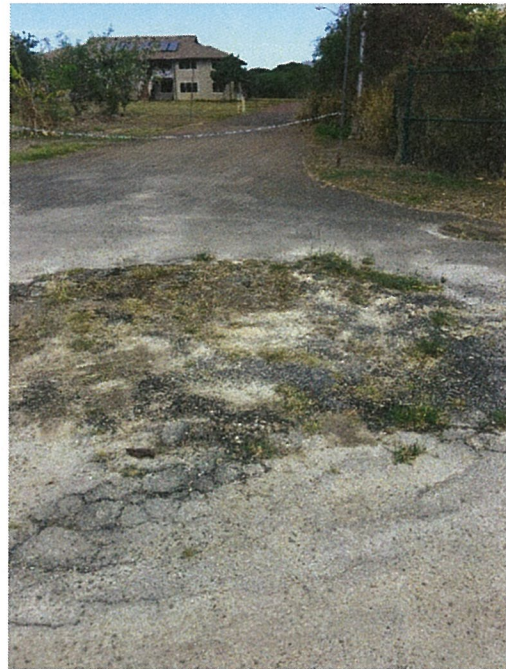
Photo 2.7. Ponding on Driveway
