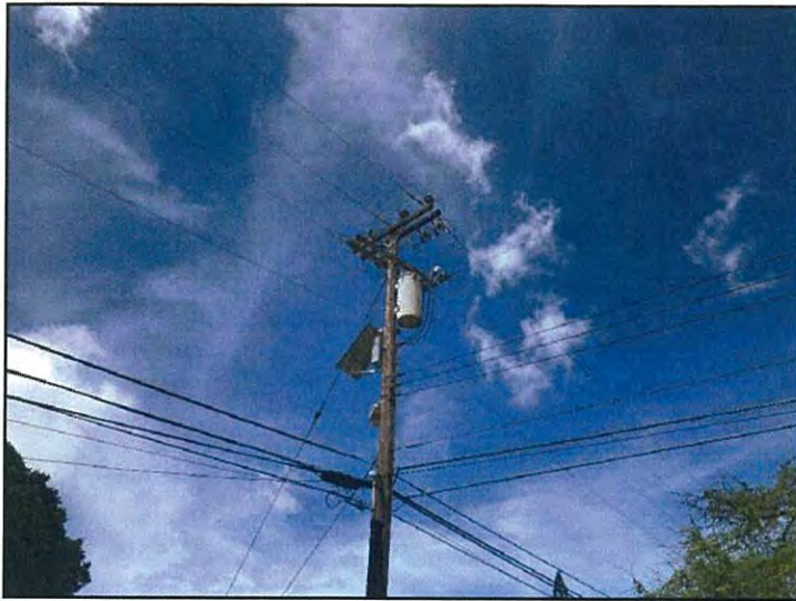
Photograph 16: View of pole-mounted transformer located north of Building No. 14 (residence).
