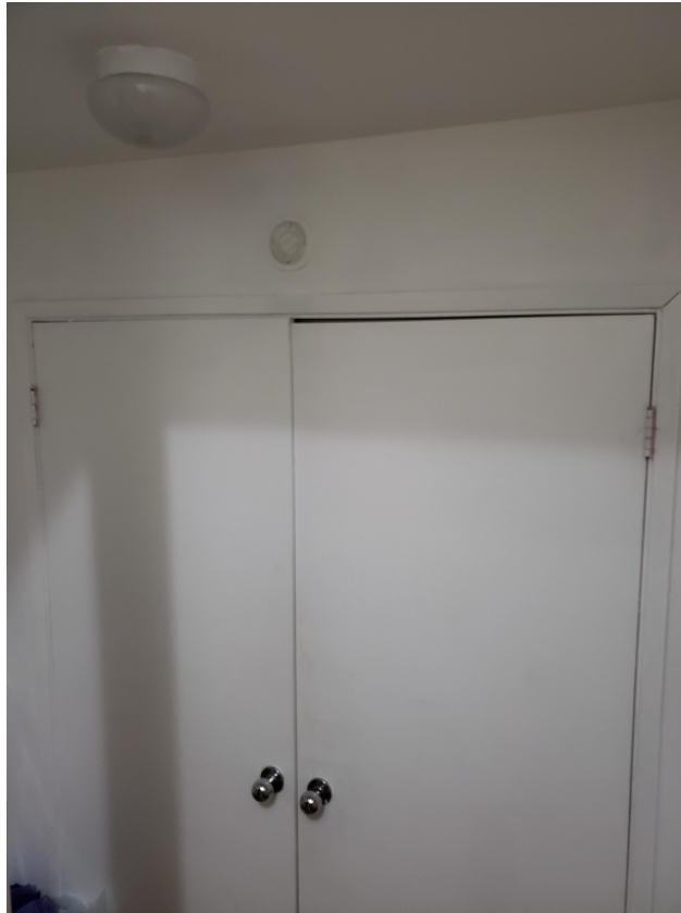
Uneven Gap and Cracked Door Moulding Interior on Lowest Level
