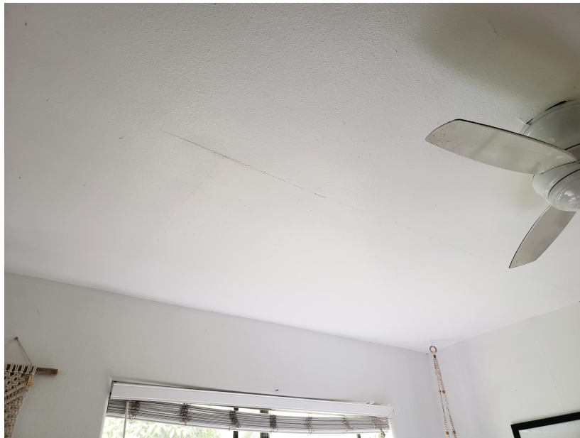
Ceiling Cracks on Lowest Level North Bedroom
