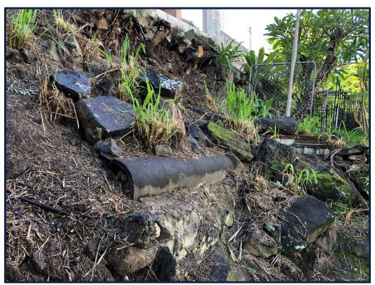
Photo No. 7 (November 12, 2020) – Central portion of slope where the abandoned concrete pipe was discovered during the previous reconnaissance. Pipe supported by grouted CRM.
