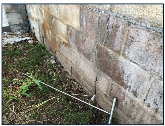
Photo No. 13 (November 12, 2020) – Additional cracks on same CMU retaining wall as previous picture. View of north side of retaining wall looking northeast.
