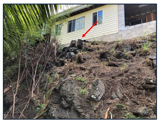
Photo No. 9 (November 12, 2020) - East side of slope. Note the loose pile of boulders stacked near the top of slope. .
