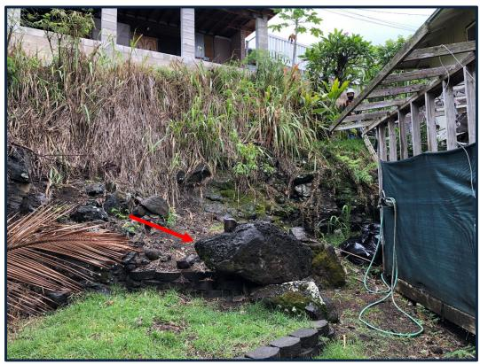
Photo No. 1 (October 23, 2020) – West half of existing slope between 440 Kauhane Street and 444 Kauhane Street. Slope is heavily vegetated. Note the 5-foot diameter boulder at the base of the slope.
