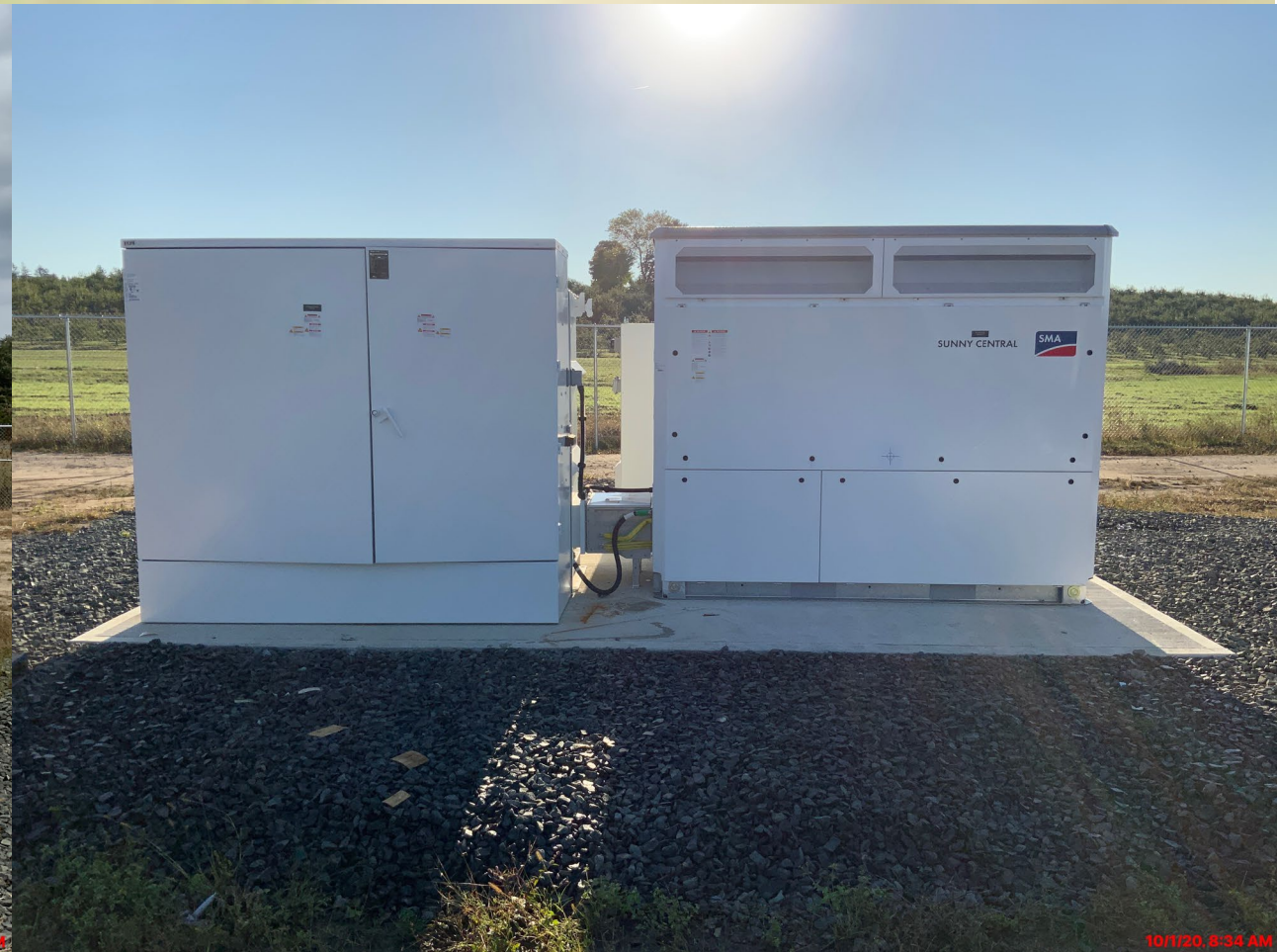
Monitoring System & Inverter
