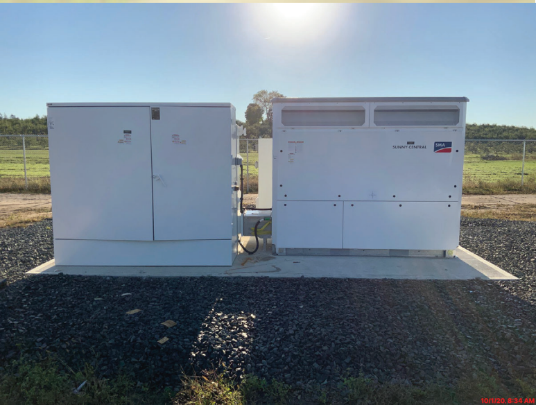
Monitoring System & Inverter
