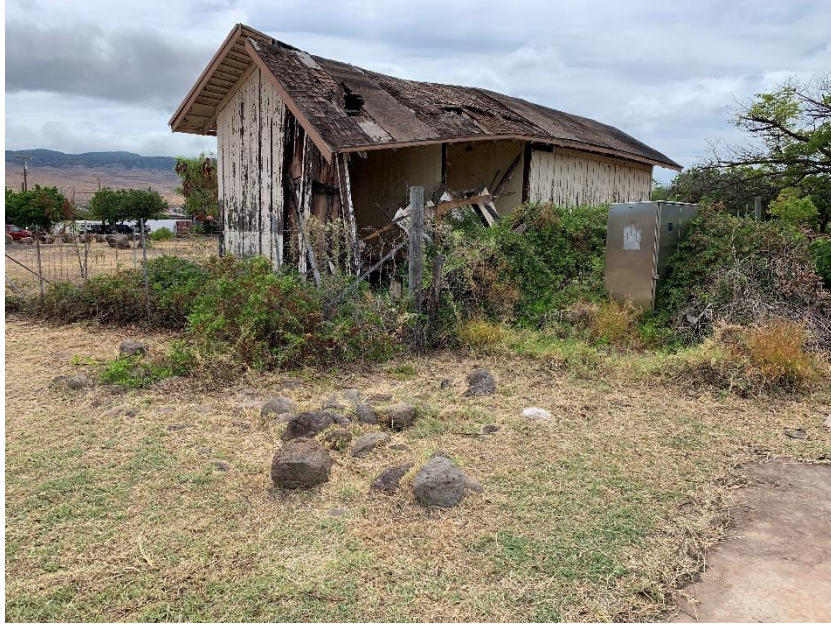
Figure 36. Makai side of the historic Kaunakakai jailhouse showing the dilapidated condition of the roof and wall; orientation is to the northeast.
