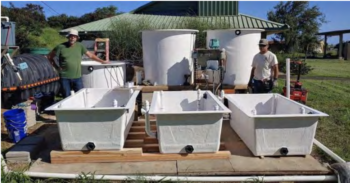
Worm wastewater treatment system at the Institute for Transformative Technologies 61
