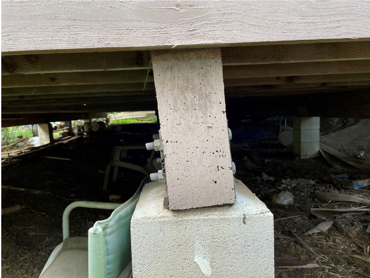
Shifting structural post
